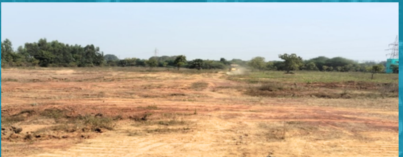
Site clearance activity- Chennai
